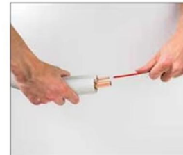
Step 1: Insert the flexible bender of the right diameter into the copper tube
