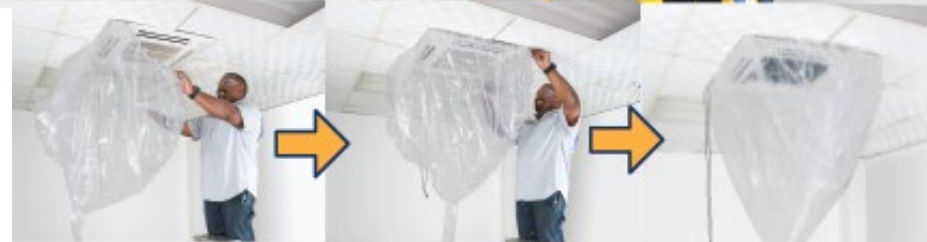
Multi-Strand Braided Elastic Collar adjusts to cassettes up to 60,000 BTU
